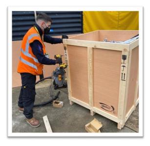
Protective timber slacks lined with Stratocell foam are used to ensure the AFM is braced and secure, reducing the risk of movement or damage.
